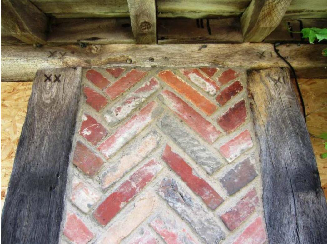
Figure 8: Detail of lean-to on west elevation, showing carpenter's marks
