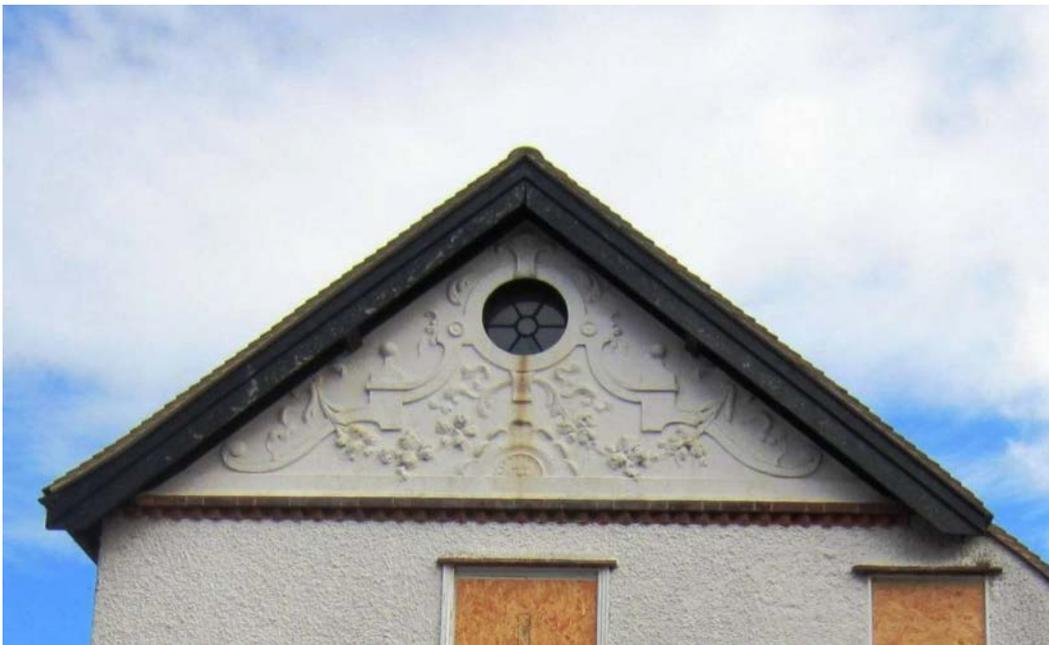
Figure 9: Pargeting in gable, west elevation
